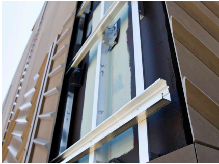
Rain-screen | Undercut Anchors
