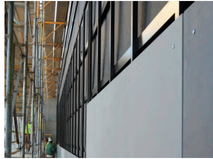
Rain-screen | Exposed Direct Fastener
